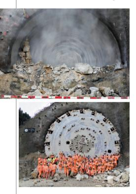
ground with claystone and anhydrite. "A nearby road tunnel, built in the 1990s had serious issues with heaving," says Grossauer. "That's why they chose a TBM to provide a closed ring which gives a stiff final lining system."
