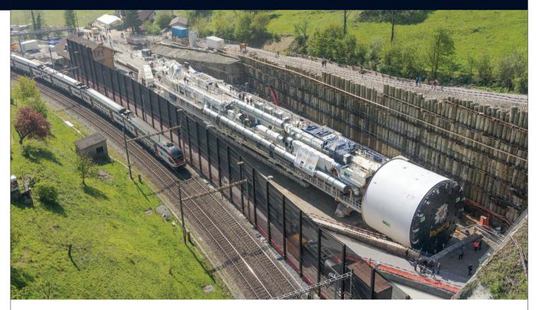
**ON 29 NOVEMBER 2017** contractor Implenia broke through on the 2.7km-long Bözberg tunnel which runs between its southern portal at Schinznach-Dorf to a northern one near to Effingen in Switzerland. The trickiest element of the tunnel build, certainly in terms of design, came at the very start of the TBM-dug section where it took over from a 175m-long traditionally constructed section.
