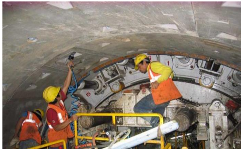
■ Fixing of bolts in segmental lining
