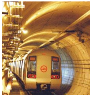
Train Passing through finished tunnel
