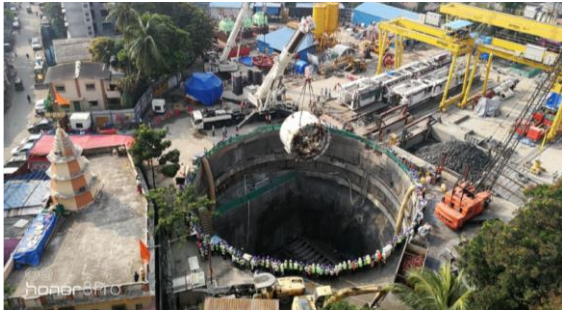
■ Aerial photo of Launching shaft construction site
