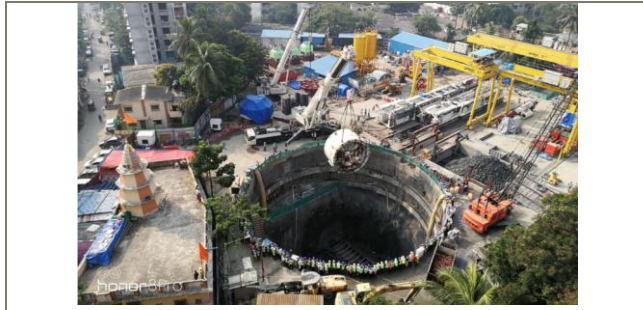
■ Aerial photo of Launching shaft construction site
