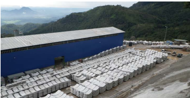
■ Installation site with segment factory
