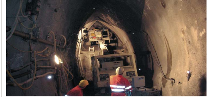
■ Shotcrete reinforcement for excavation new tunnel
