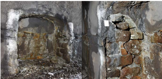
■ Old tunnel, deteriorated sections and brick lining
