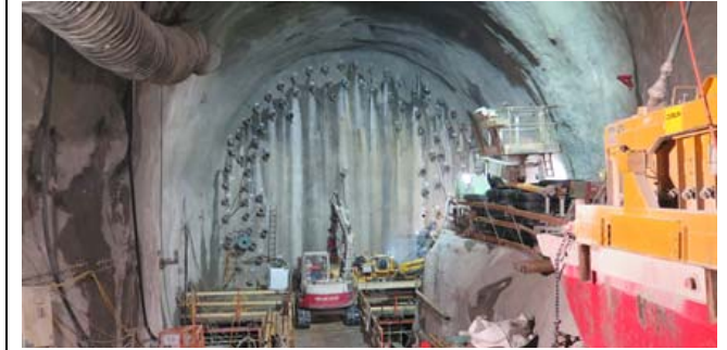
Freezing tubes at cavern at Tm 1'300
