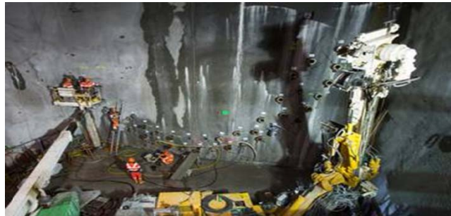
■ Securing of the new portal area
