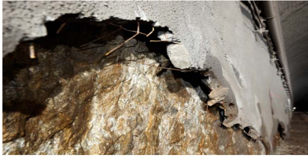
Deteriorated area at the vault section of old tunnel
