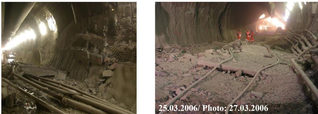
Fig. 9. Single-track tube east/north. Left: damage of the shotcrete support after the M1.9 event. Right: invert failure and bulking after the M2.4 event.
